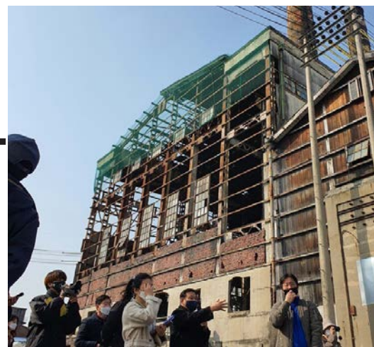
Existing Power Plant building
