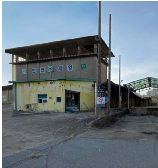
Existing factory tower
