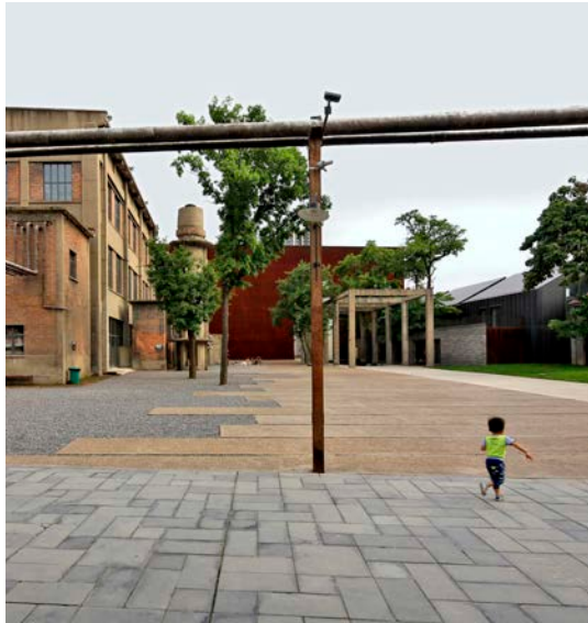
Preserved industrial structures ref.: Xi'an Dahua Textile Mill by CADG
