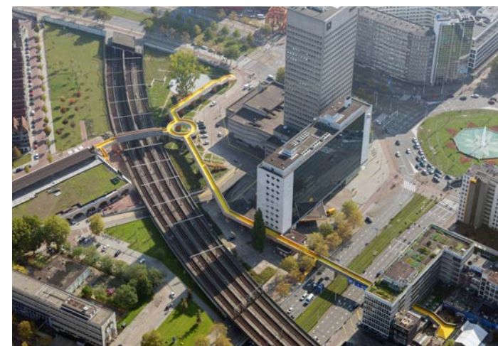
Elevated Walkway The Luchtsingel / ZUS / Netherland
