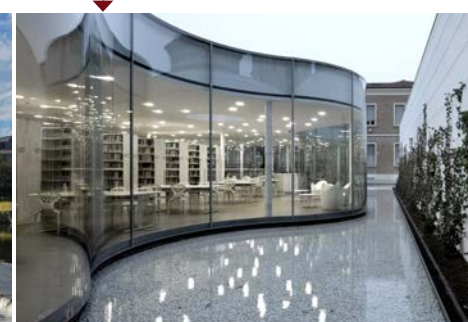
Curved Facade Reference
